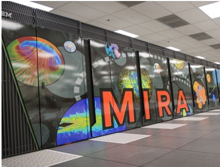
Leadership HPC Facility
